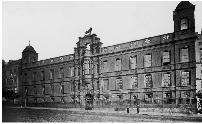
Northumberland House prior to demolition in 1874.
